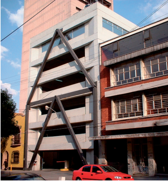
FIGURE 4-2 Mexico City parking garage with external steel frame retrofit. (Source: Author.)
