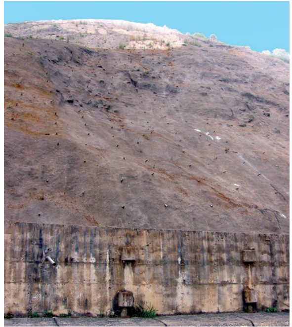
FIGURE 4-5 Slope covered with concrete and outfitted with drainage pipes to prevent landslides. (Source: Author.)
